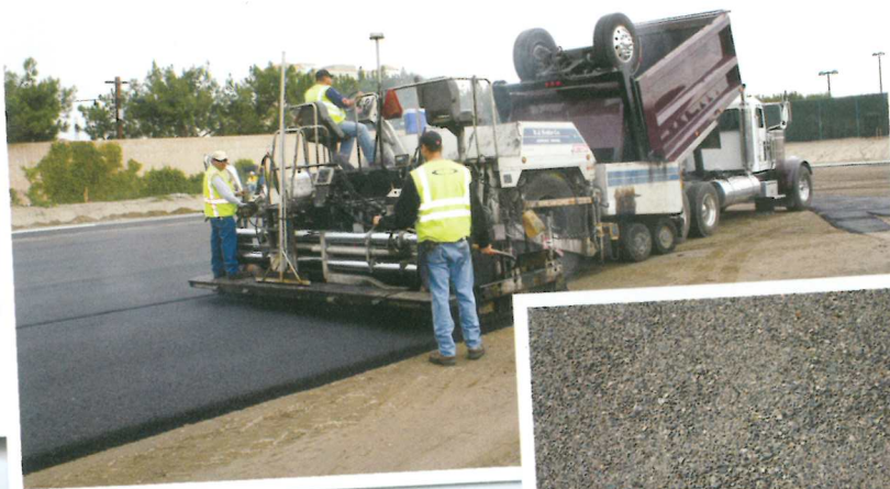
(Below Left) Porous asphalt manufactured by R.J. Noble Company contains little sand or dust with an interconnected air void space of approximately 16% compared to 3% to 5% with conventional HMA.
