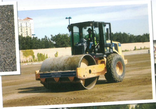
(Below) Compacting subgrade prior to paving.
