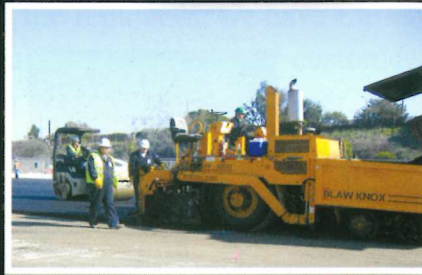
Blue Diamond Materials - Continues EcoMat® Advancement at Exxon Refinery in Torrance
